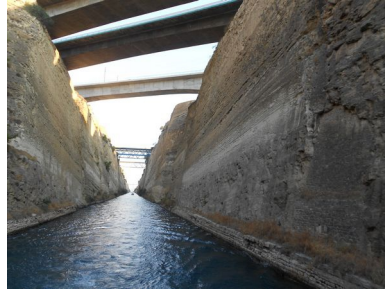
The old and the new, Bridges over the Corinth
