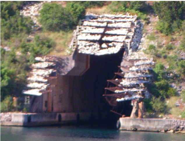
The grating covered with rocks are designed to swing open
